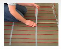
We do not advise taping over the entire length of wire, as it can create unnecessary air pockets around the heating wire.
