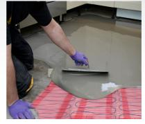
we recommend a minimum of 8mm suitable latex levelling compound to cover the heating mat/cables to ensure even heat distribution.
