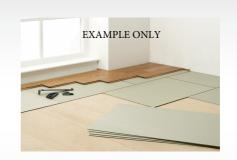
(**DO NOT** use XPS insulation boards on wooden sub-floors)
