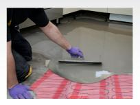
If you are using a suitable vinyl/ carpet or engineered/laminate floor as the final covering then we recommend a minimum of 8mm suitable latex levelling compound to cover the heating mat/cables to ensure even heat distribution
